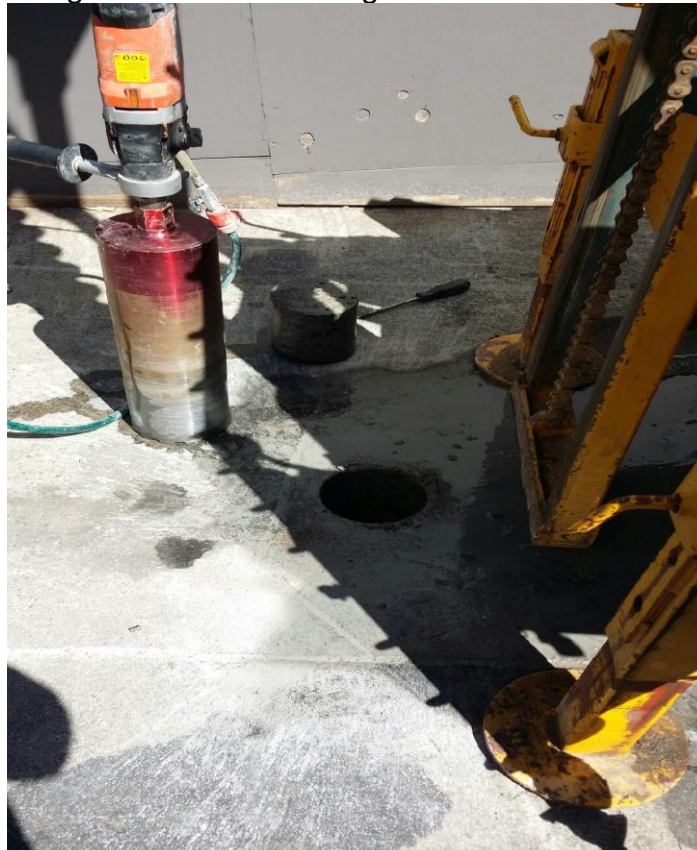
Image 4: Concrete Coring Borehole Numbered 1
